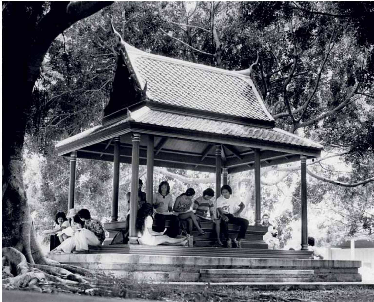
A traditional Thai sala (pavilion) provided a setting for sociable gatherings or quiet meditation for nearly 30 years. His Majesty King Bhumibol Adulyadej of Thailand donated the original in 1967 and, in 2006, sent artisans to build a new one.
