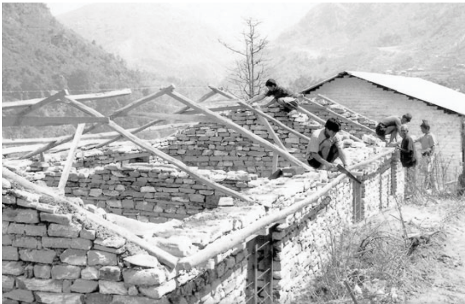
A Room to Read project school under construction in Nepal
