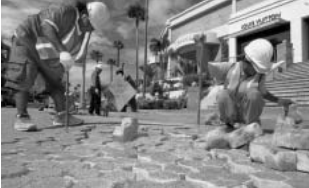
Workers fix the brick crosswalk in front of DFS Galleria in Tumon. Photo: Pacific Daily News
